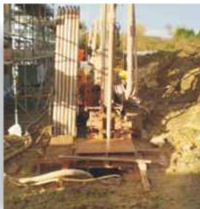
Installing the ground source heat pumps at Chorley
